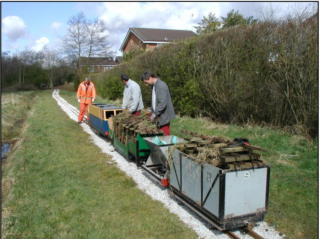
Engineering works on the HMR on 27 March 2008. The section of line at this location was realigned during the winter of 2007/8 and new track was laid. The original track from the early 1980s was being removed from site by a works train. Photo by Paul Wright
